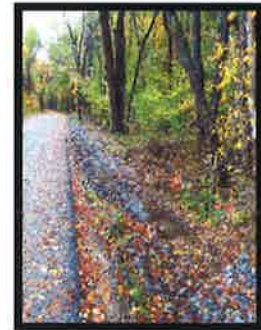
Creek Road Project above Lake Wilhelm in New Vernon Township
