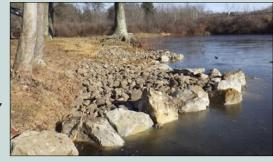
Lake Management Society grant to protect the shoreline in this heavy -use area. Those triangles of rock are called stone deflectors and are used to stabilize the shoreline and reduce sediment into the lake.
